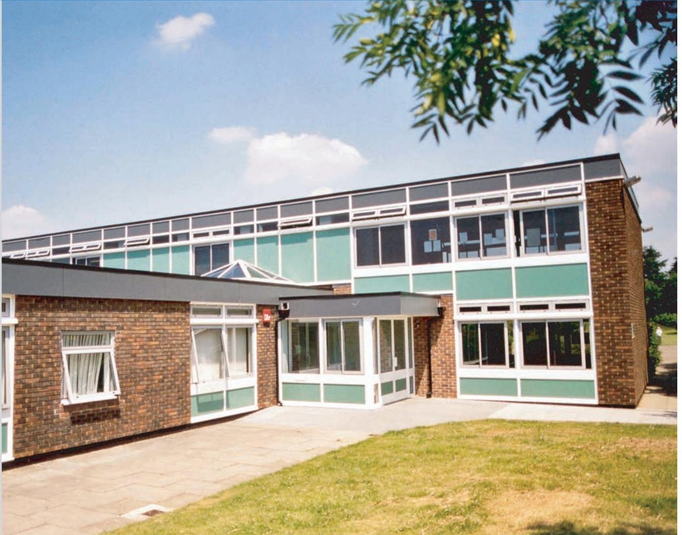
This project was completed in February 2003 and was a refurbishment of a typical 1960's timber panelled façade. On such projects a close match to the original building is a priority. Comar 2, the cost effective alternative to curtain walling, offers an excellent solution. Two mullion widths are available: 35mm and 45mm with high span options that ensure that single and multi-storey options can be completed with the same slim sight lines.
