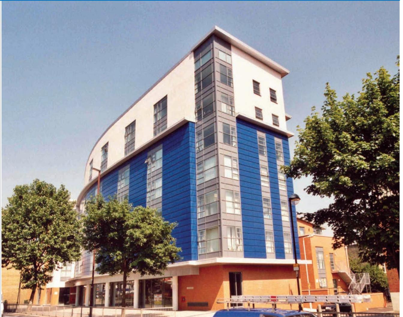
The design of the envelope using different textures and façade materials resulted in this eye-catching development. Creative use of aluminium provided the glazed façade, whilst blue rain-screen paneling created texture into insulated rendered brickwork.
