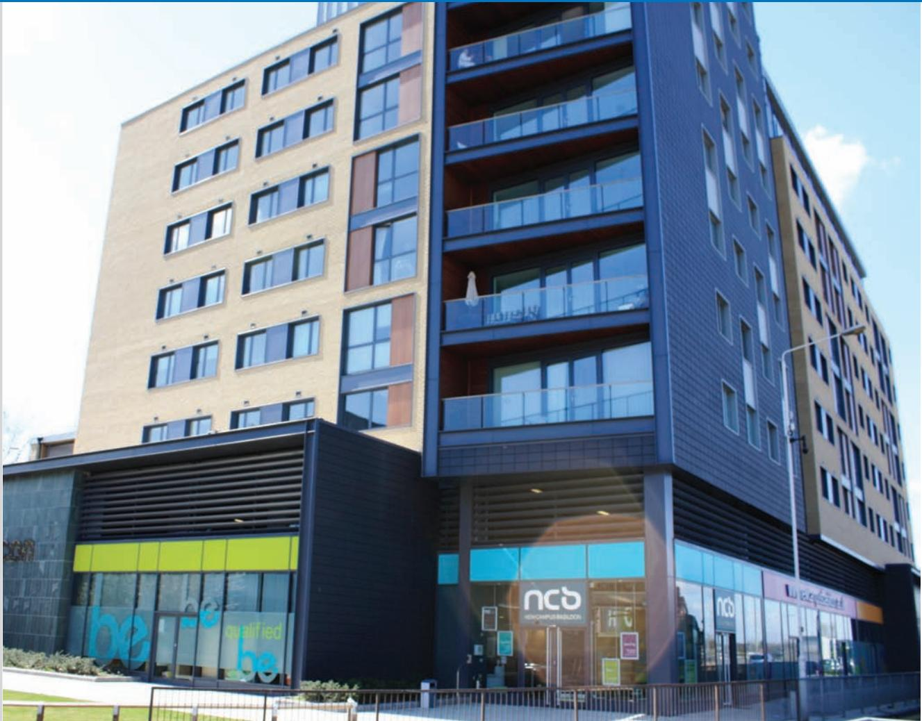
Comar Architectural Aluminium Systems and Hollybrook Construction supplied Comar 2 window walling, Comar 5P.i thermally broken windows, Comar 6 curtain walling, Comar 7 and 7P.i doors and Duco louvre blades for a new build mixed use development, comprising of retail units and apartments, in Basildon, Essex. The retail units have been 'let' to New Campus Basildon (NCB) which forms part of the Essex University facilities.
