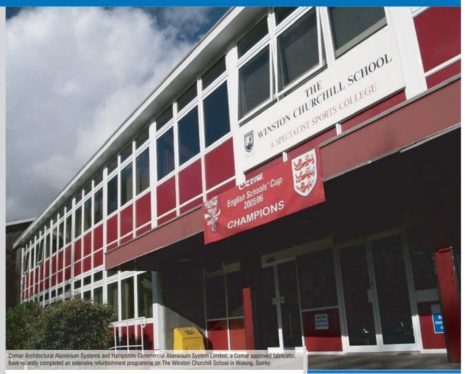
One of the elevations consists of a two-storey, 200m span of cladding, originally timber, which had reached the end of its life cycle. To totally update the building Comar 2 window walling was specified with integrated top-hung opening vents and panels. Comar 2 offered a precise fit to the specification requirements of the building, offering fast-track installation, a wide range of glazing options, integration, security, high-span mullions and transoms
