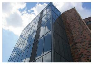
For facetted curtain walls, corner mullions are adjustable from 15° to 145° in Comar 6 and from 7.5° to 165° in Comar 6EFT. This means that roof-glazing applications, such as barrel vaults, pyramids and sloped glazing, can be achieved.
