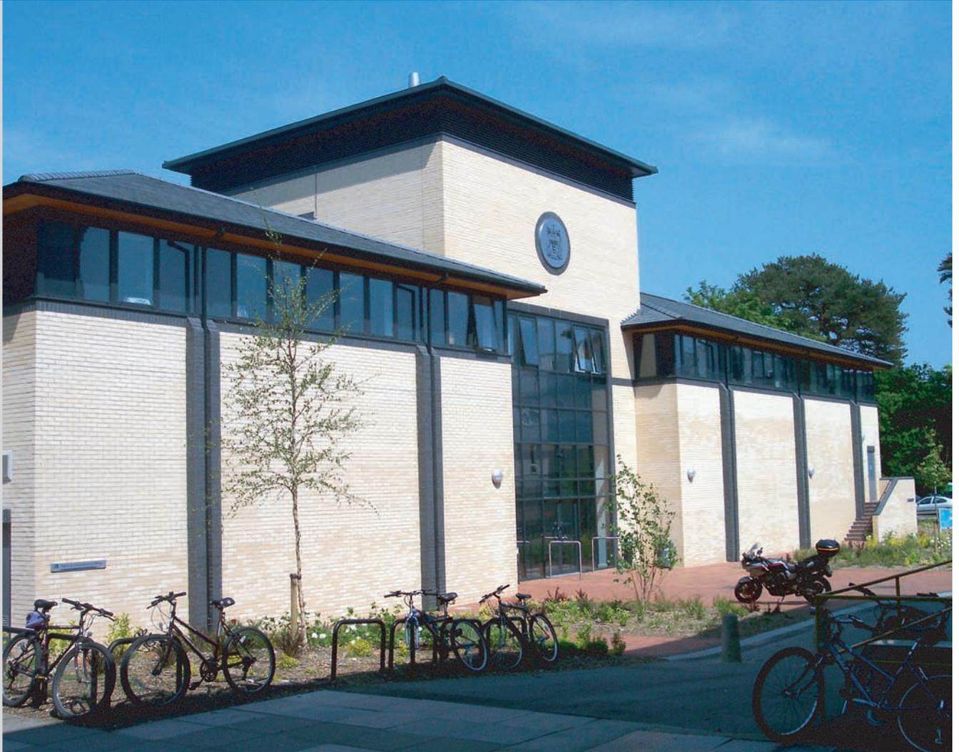
This stunning project was created with the use of contrasting sandstone brickwork and black polyester powder coated architectural aluminium. This was a new-build project and the symmetry of the building created the clean lines of the project. Comar 5 top-swing windows were used in a ribbon configuration and were tinted to reduce glare.
