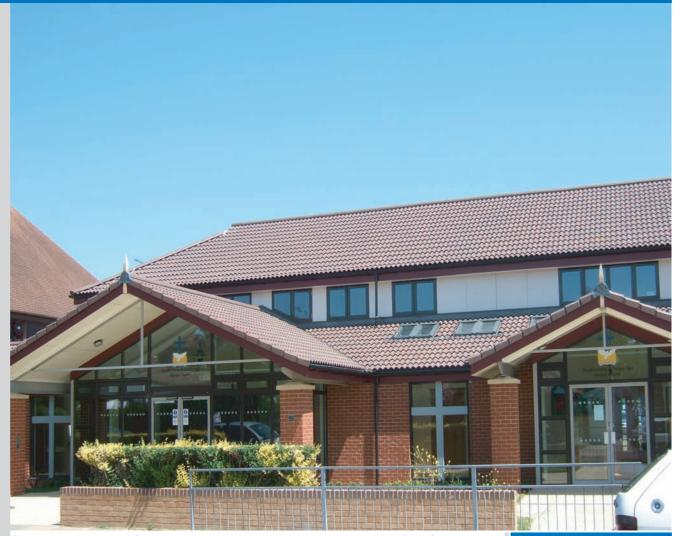
Comar Architectural Aluminium Systems, with their approved fabricator Anglia Fixing Limited, supplied Comar 2 Window Walling, Comar 5P.i Windows and Comar 7 Swing Doors for a new build church. A key requirement for this project was that the glazing featured an imposing cross design within a number of different units.
