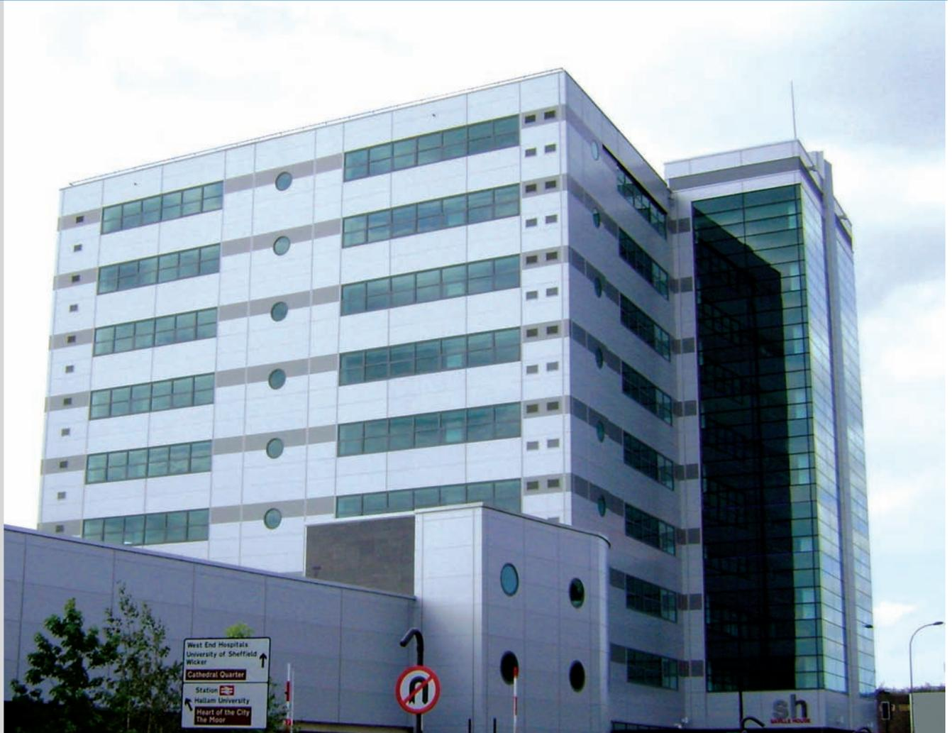
Comar Architectural Aluminium Systems and their approved fabricator, APIC (U.K.) Ltd., was specified by Archial Architects to undertake the multi-cladded office development, Saville House in Sheffield, using aluminium glazed facades solutions from Comar and Eurobond cladding panels.
